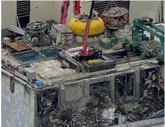
Unit 4 after the hydrogen explosion. The bright yellow object is the lid of the Reactor Containment Vessel.
